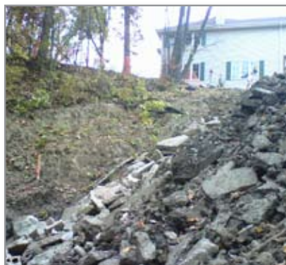
Erosion caused by stormwater runoff threatened nearby homes.
