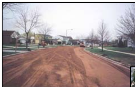
Thompson under construction
